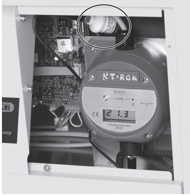
Fig. 7.3: Replacing the oxygen sensor
